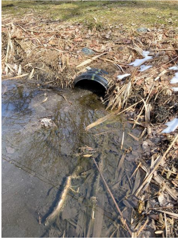
Above: Outfalls near Spring Ave East fill with sediment quickly (March 2023)
