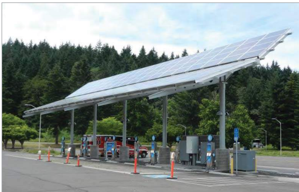
Solar canopy with EV supply equipment
