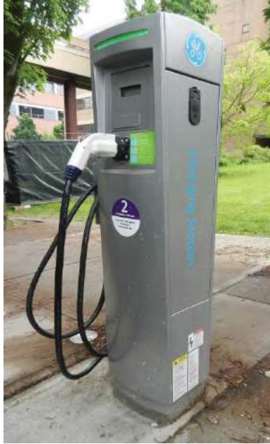
Level 2 EV supply equipment
