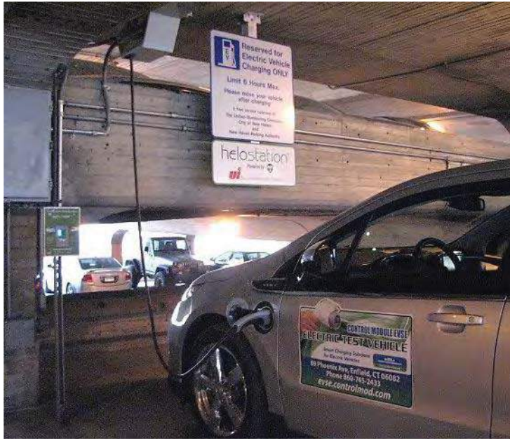
Level 2 EV charging cable automatically lowers from ceiling (photo courtesy of EVSE Ltd.)
