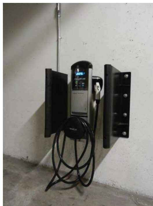
Wall-mounted barriers offer an alternative to wheel stops and bollards
