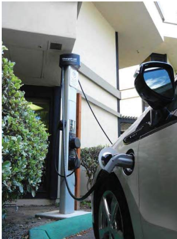
Level 2 EV charging cable retracts
