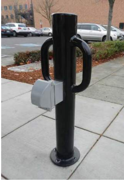
Level 1 EV supply equipment
