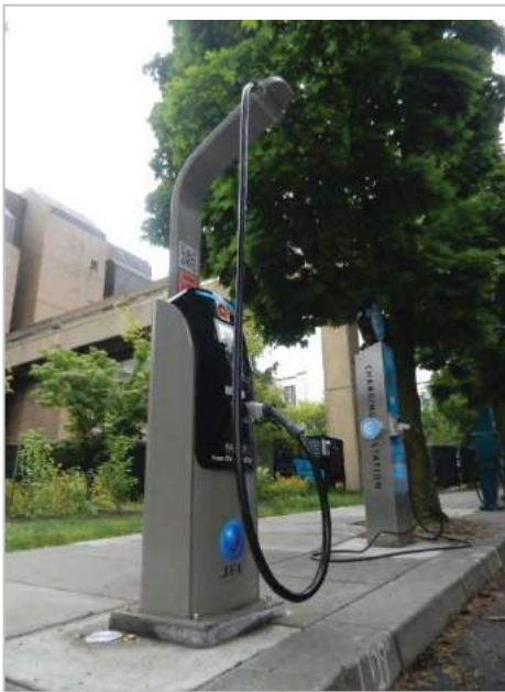
Suspending cable assists with handling
