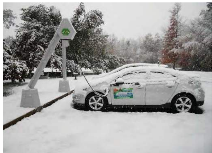
Suspended, retractable cable prevents the cable from being buried in snow or ice (photo courtesy of EVSE Ltd.)
